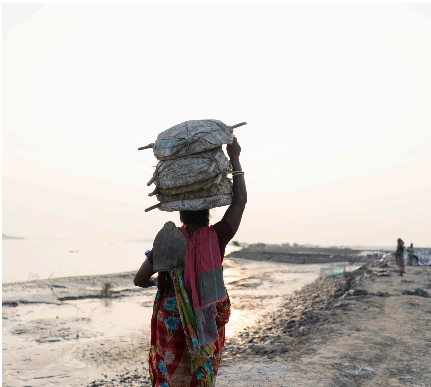
A woman on her way to repair the damaged embankment in Munshiganj, Shyamnagar. Photo: Abir Abdullah/GTS
