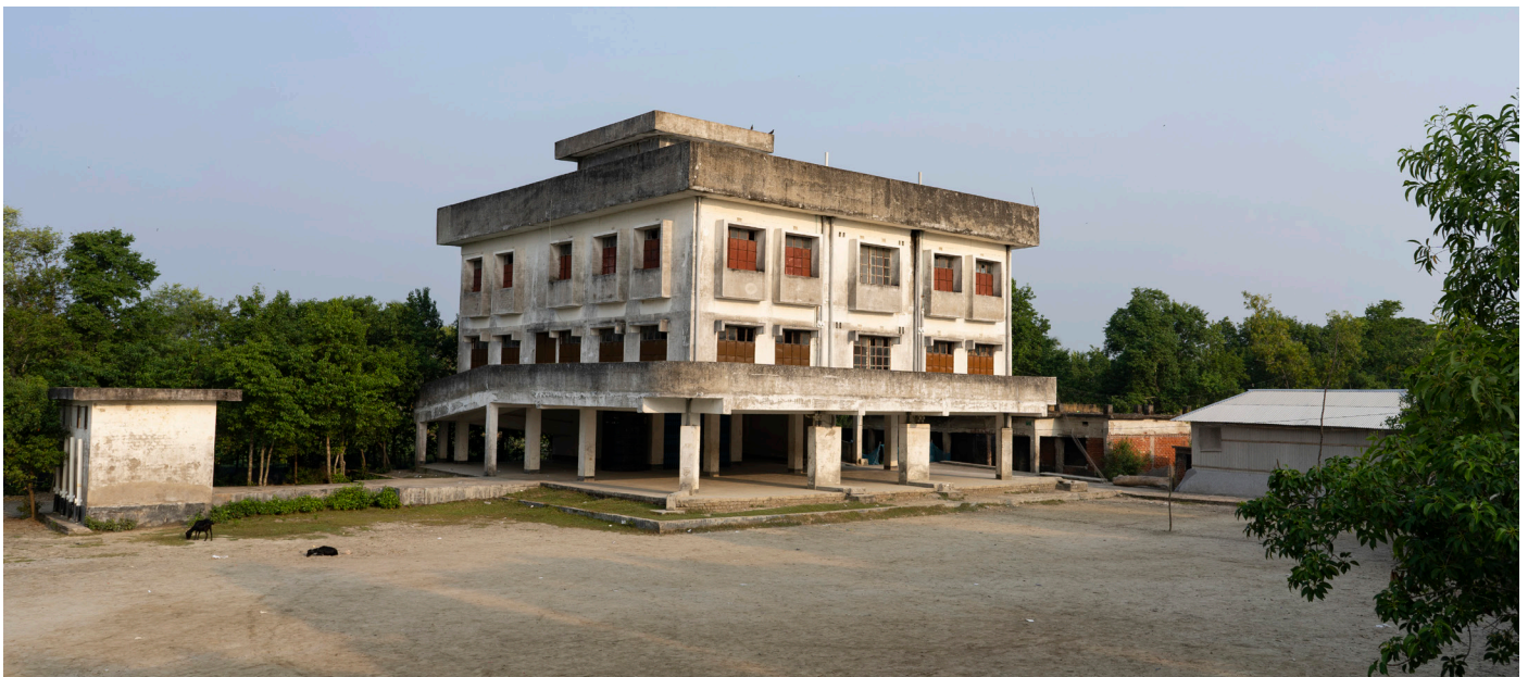
A school-cum-cyclone shelter in Parakatta, Munshiganj, Shyamnagar. Photo: Abir Abdullah/GTS
